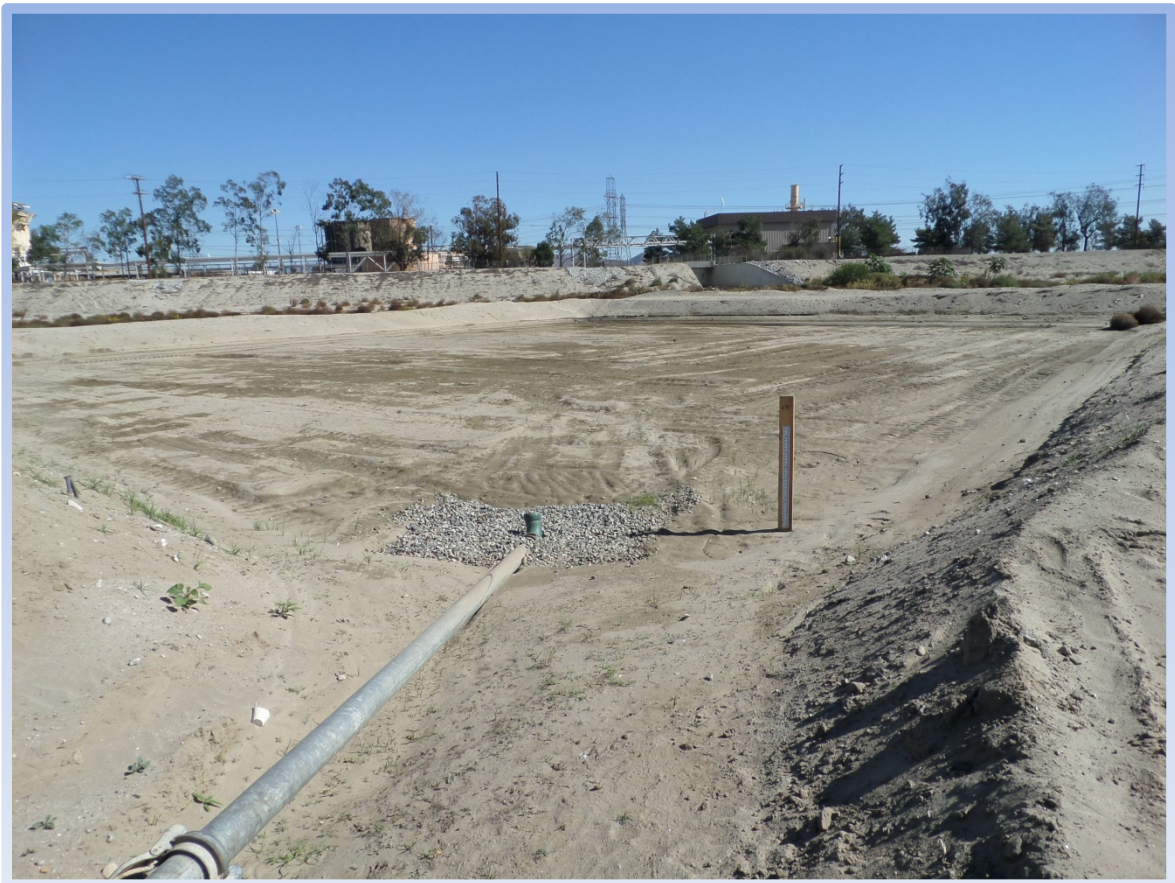
Figure 7: Typical PTC Inlet and Staff Gauge
